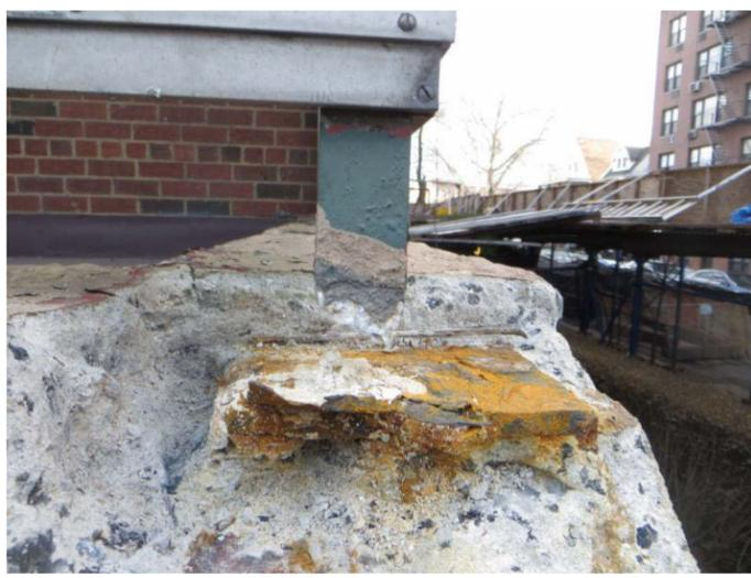
Building managers should monitor the transition between railing materials. When dissimilar metals come into contact, a galvanic reaction may occur, causing the metals to corrode. For example, an aluminum railing that is anchored directly to structural steel will likely deteriorate when exposed to air and moisture...[Read more](#)
